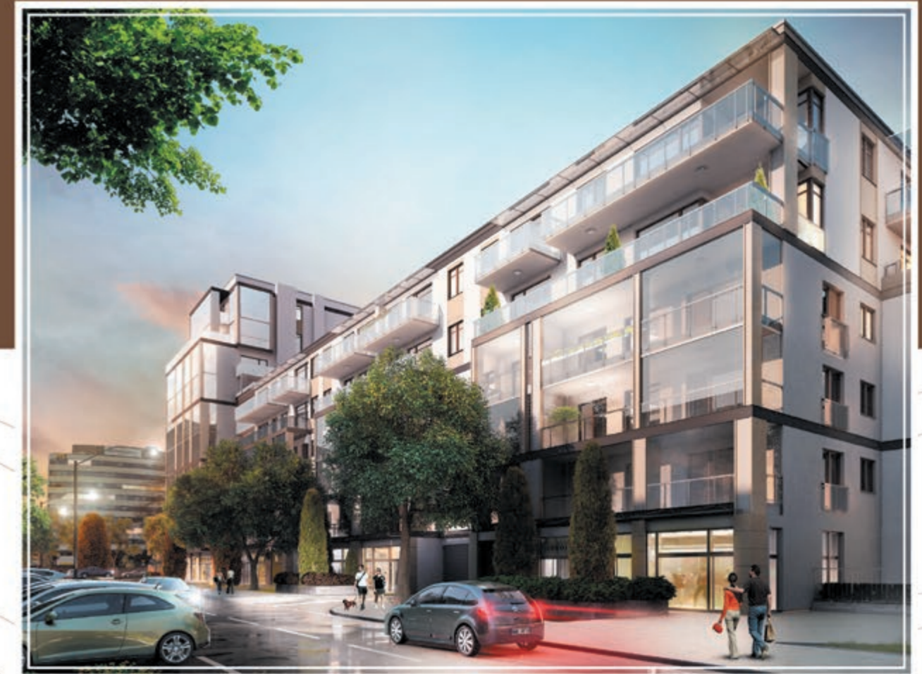
VIEW OF THE RESIDENCE FROM NARUSZEWICZA STREET
