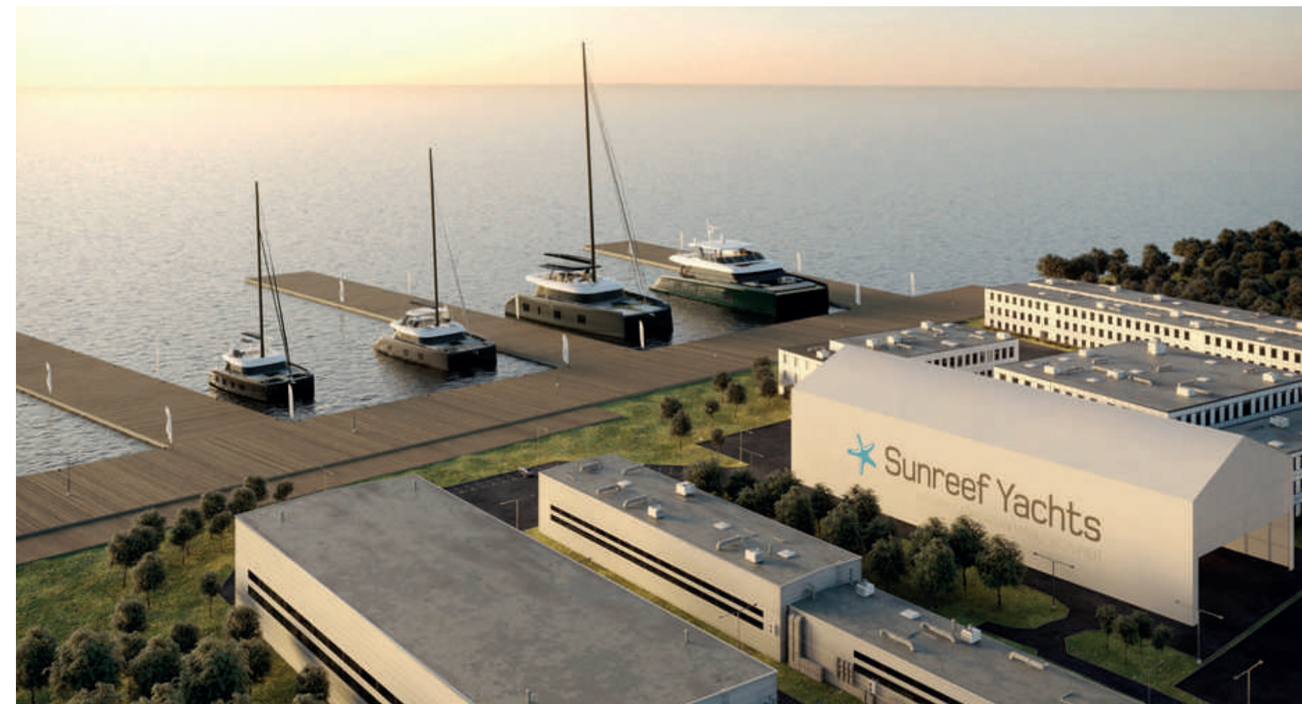
After almost two decades at the historic Gdansk Shipyard, Sunreef is moving to a new 80,000sqm site (below) beside the Martwa Wisla river
